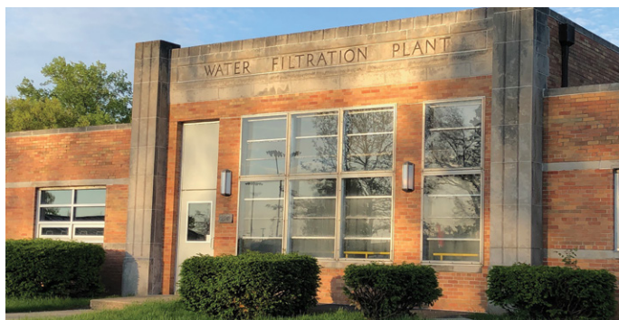
Water Treatment Plant 1 in Lincoln Park, opened 1950.
